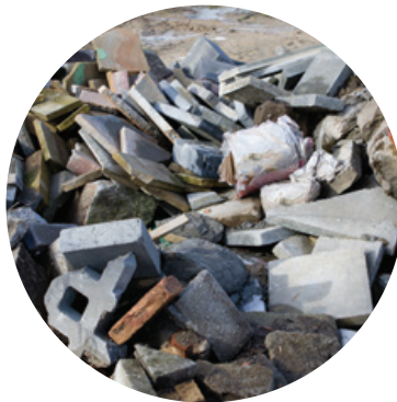
MIXED CONSTRUCTION AND DEMOLITION WASTE
