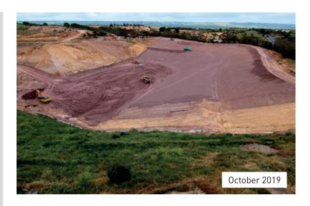
Onsite crushed shale is utilised to prepare the processed mineral baseliner and sideliner layer.
